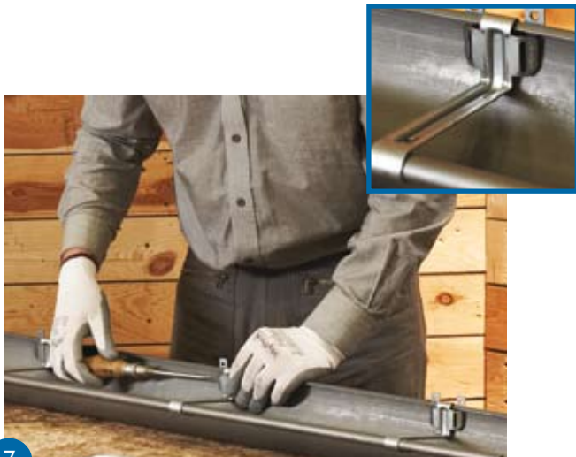
7 Secure each bracket to the gutter by folding over the 2 tabs.
